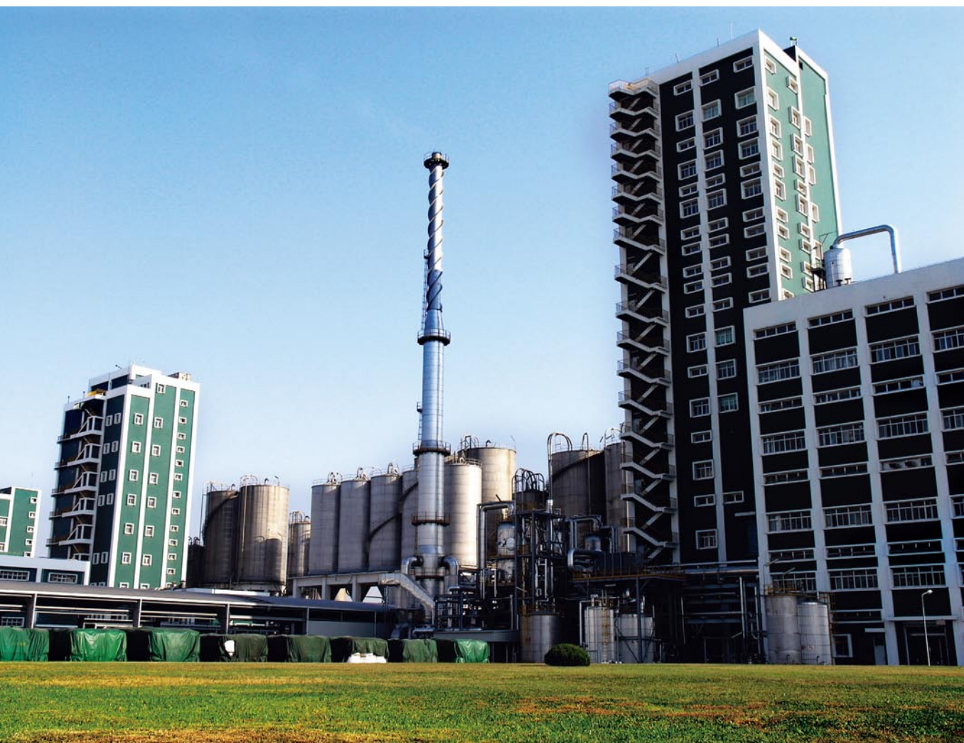
■ Far Eastern Industries Shanghai Plant, China
